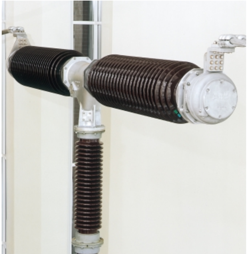
A DOIT current transformer mounted on a 420-kV circuit-breaker of type HPL 9
