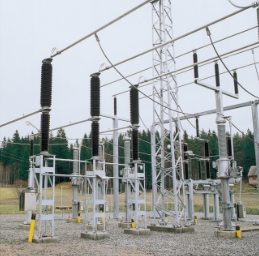
The LTDS-Compact gas-insulated disconnecter also serves as a post insulator.
