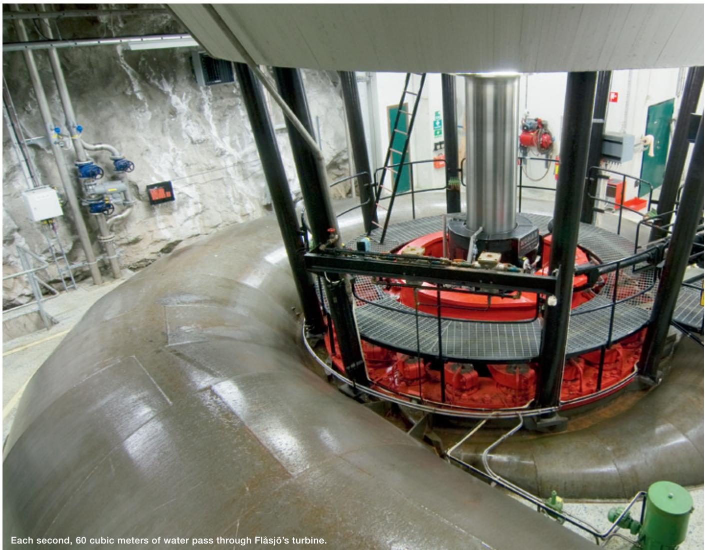
Each second, 60 cubic meters of water pass through Flåsjö's turbine.
