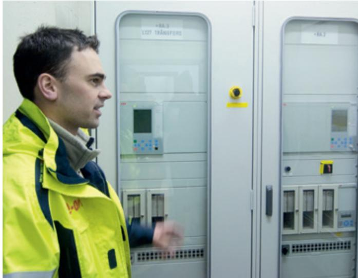
The outgoing high voltage grid line from Flåsjö is protected by REL670 relay protection.
