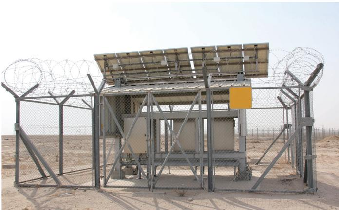
RTU in a natural gas multi-well PAD application
