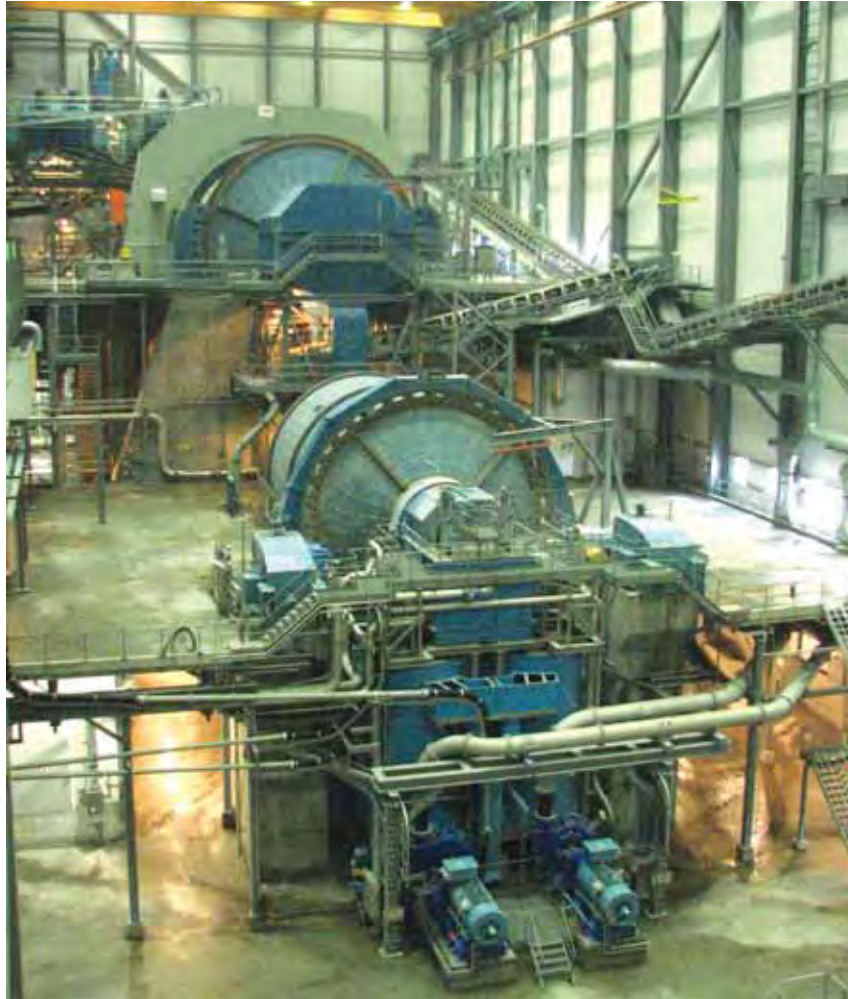
A key element of Boliden's ambitious expansion program for its Aitik copper operation is the new concentrator. Shown here, at rear, is one of the plant's 2,200-mt/h autogenous mills, the largest of their type in the world. The concentrator's two AG mills, supplied by Metso, are powered by 22.5-megawatt ABB gearless drives.
