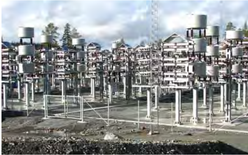
ABB installed a large array of harmonic filters, shown here, to lessen the impact of the mine and mill's high power demands on the local electrical grid.
