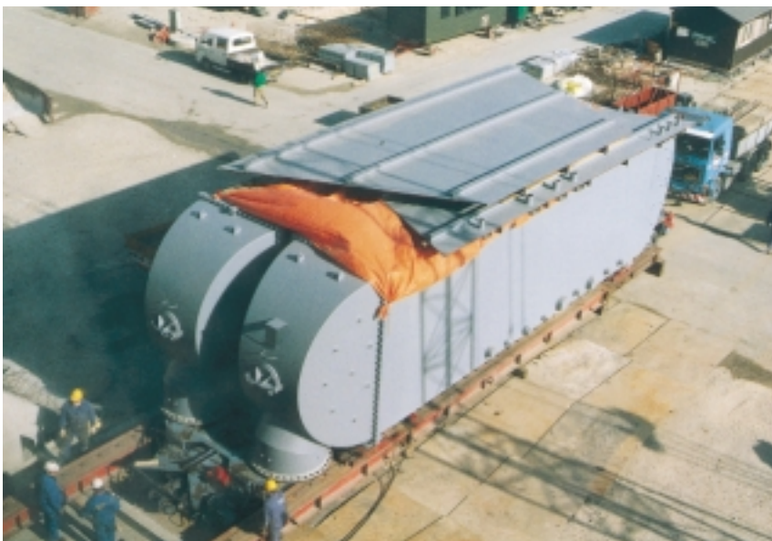
Two CM/H condenser modules ready for installation on the site of the 320-MW Avedøre 1 steam power plant in Denmark
