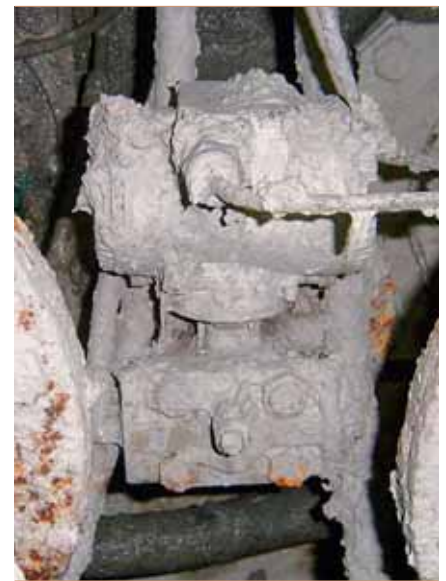
2 Harsh environment with high risk for plugging
