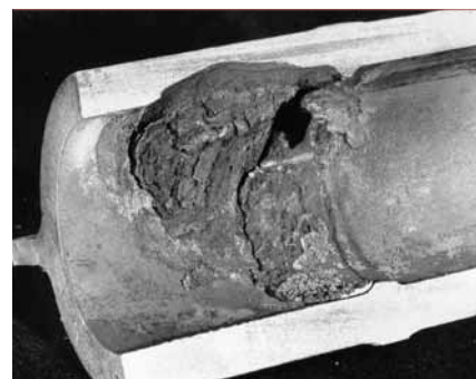
2 Tube weld corrosion due to poor control of chemical conditions in steam-water cycle
