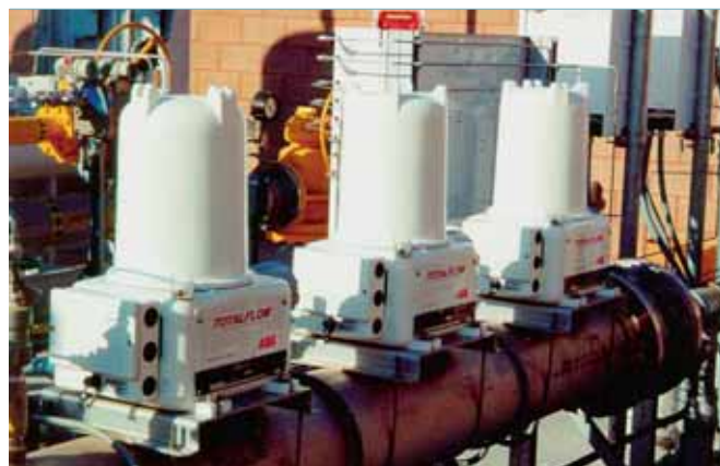
3 Energy metering and blending system based on ABB Totalflow natural gas analyzer
