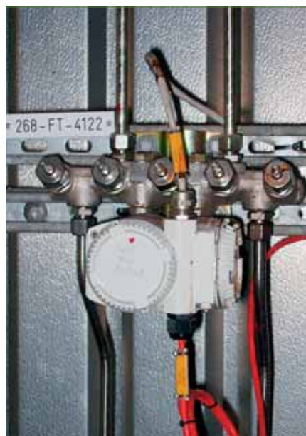
1 Installed multivariable transmitter
