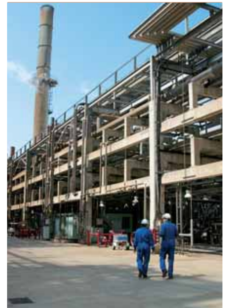
1 A typical plant can have hundreds of pressure transmitters installed
