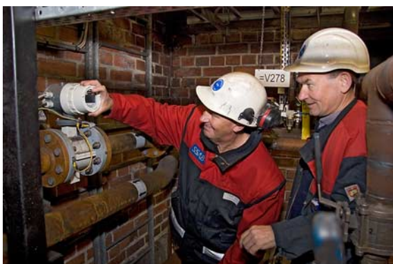
Björn Olsson was part project manager for the electricity and control part at the renovation of the blast furnace, while Hans Holgersson had the responsibility for the construction of the instrument circuits. Here they are controlling a inductive flow meter from ABB that measures the cooling water temperature in the furnace.
