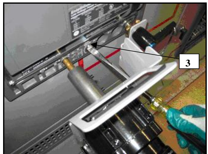
Fig. 3 Opening Racker access door
