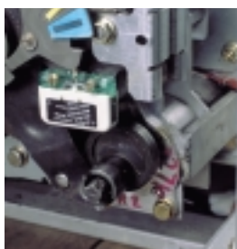
Spring charging geared motor.
