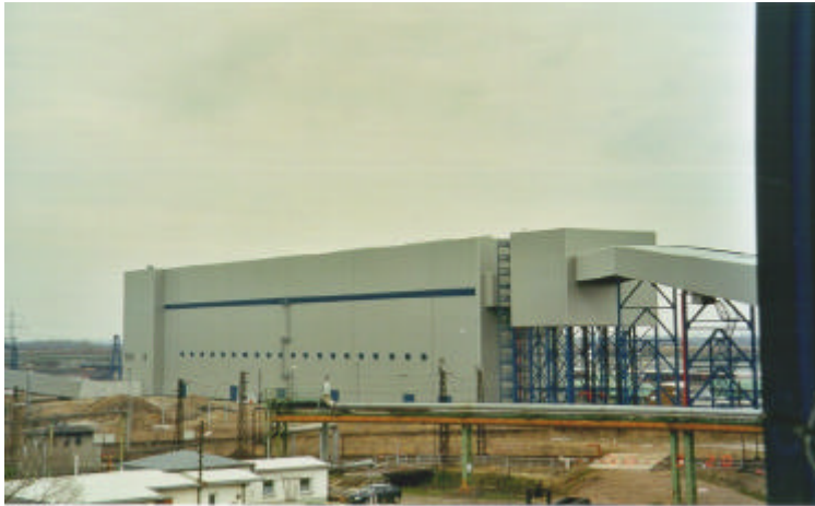
Stand-by lignite bunker in power station area
