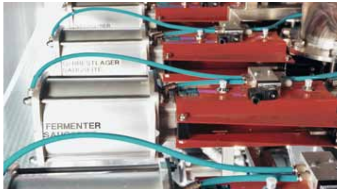
The ABB Freelance process control system controls the complex systems engineering of a modern biogas plant and ensures maximum gas output at a constant quality.
