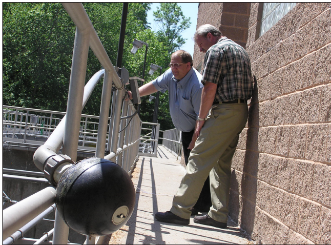
Figure 3: Howarth and Tim O'Dell, Assistant Superintendent, Swivel the DO Ball Sensor into the Air to Calibrate the System Based on the Air Saturated Oxygen Level.
