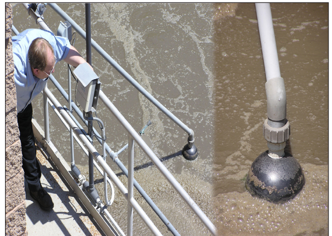
Figure 2. Dissolved Oxygen Sensor and RTD Sit Flush with the Bottom of a Large Floating Ball. Wastewater Flows Passed the Ball, Keeping the Sensors Free of Debris. Superintendent Mark Howarth Checks DO Reading on Nearby ABB Transmitter. The Transmitter Compensates for Temperature and Elevation and Sends a 4 To 20 MA DO Signal To The Control Room.
