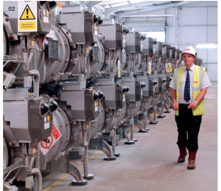
01 Port Ham's old AIS in the foreground and new indoor GIS indoor substation | 02 Twenty bays of switchgear are housed indoors
