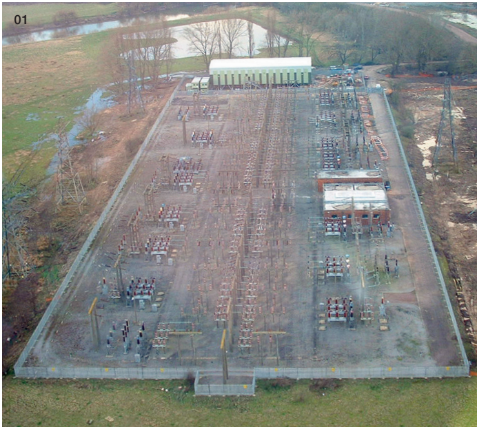
01 Port Ham's old AIS in the foreground and new indoor GIS indoor substation | 02 Twenty bays of switchgear are housed indoors
