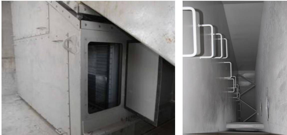
Figure 3 Access door and ladders inside the motor
