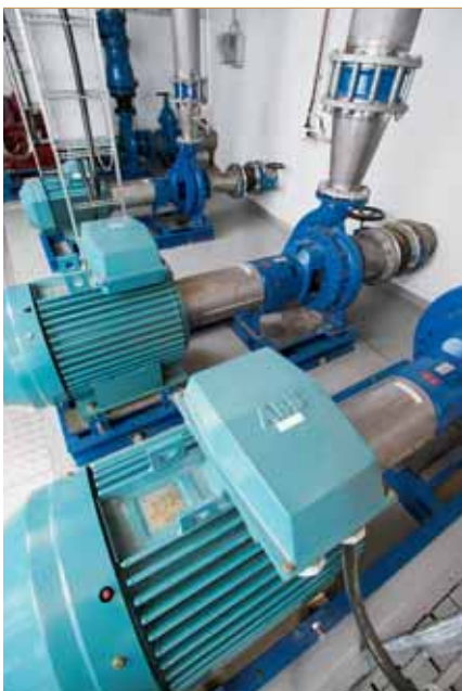
A pressure-boosting station (Pietersaari Finland). The drives are equipped with DTC and intelligent pump control (IPC)
