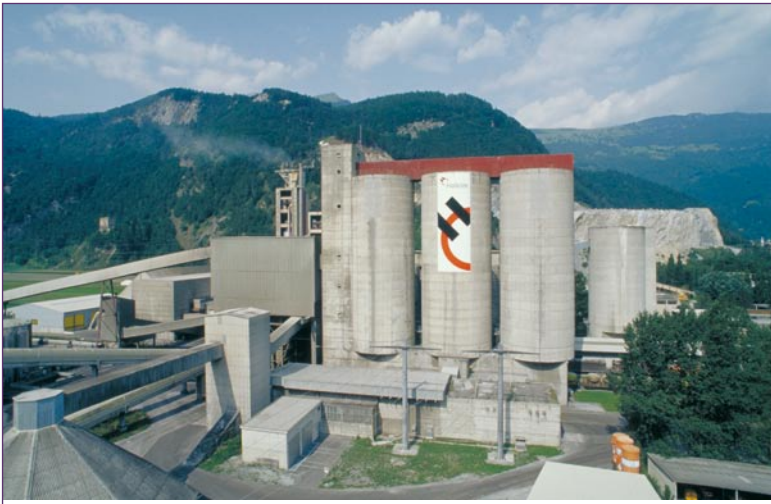
Figure 1. Holcim's Untervaz plant.
