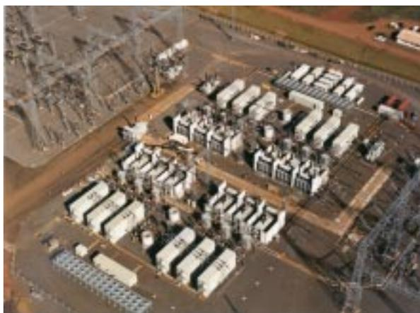
Fig.1 Overview of the 1100 MW modular back-to-back HVDC station in Garabi, Brazil.
