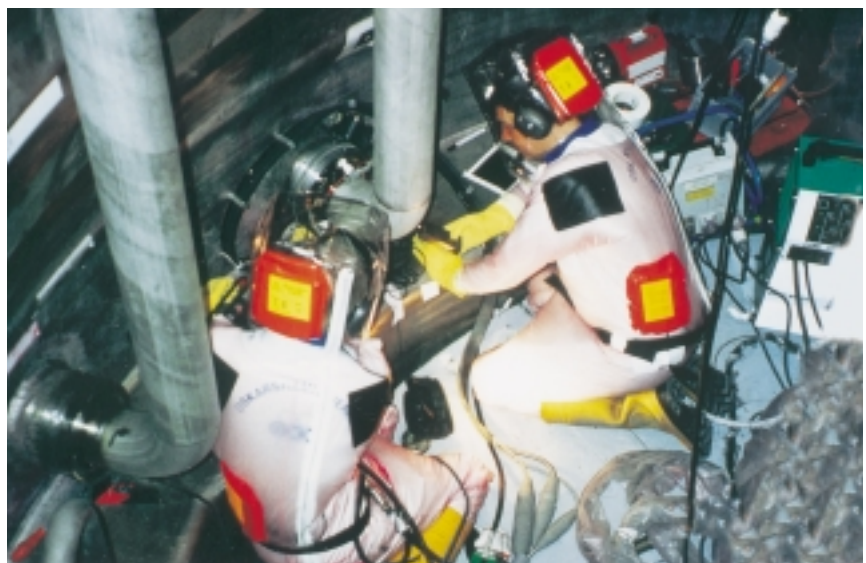
Welding feedwater pipes in the reactor pressure vessel 5
