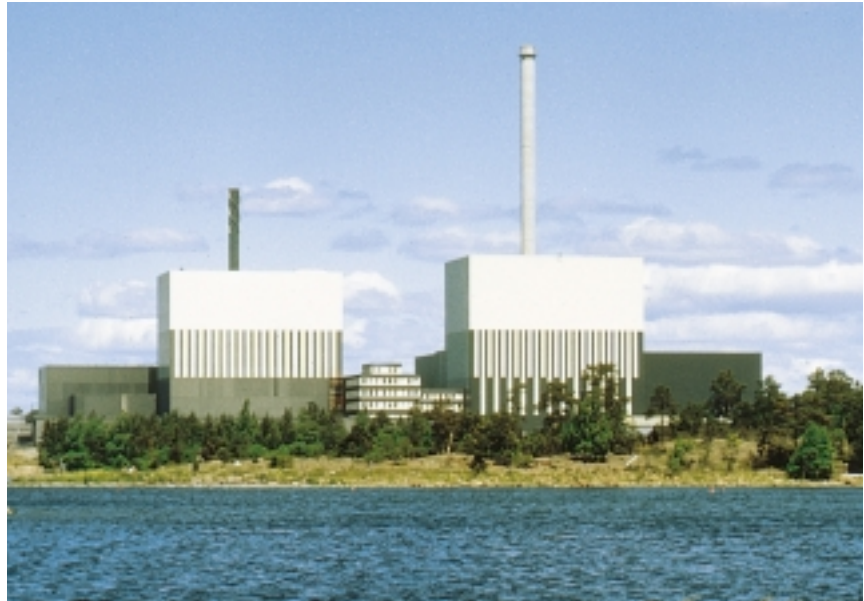
Oskarshamn nuclear power plant on the Baltic Sea coast. Oskarshamn 1, Sweden's first commercial nuclear facility, is on the left. The plant, from ABB Atom, began operating in 1972 and today exhibits a net electrical output of 440 MW. 1
