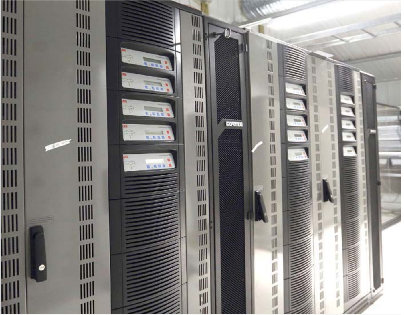
ABB's modular UPS system ensures the reliability of the data center power supply and perfectly supports the customers need in terms of scalability and flexibility
