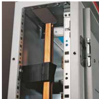
Cabling control is made easier thanks to lateral removable panels
