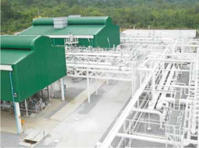
Saiyok Gas Compressor Station, Thailand for PTT
