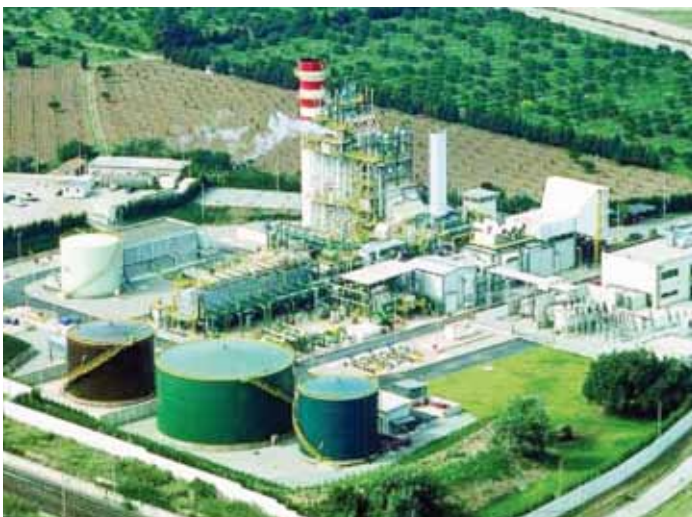
Milazzo Combined Cycle Power Plant Italy for Sondel
