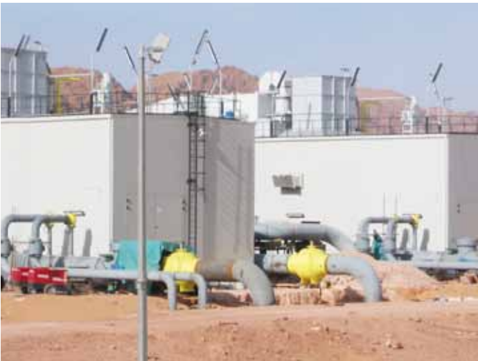
Hassi R'Mel Boosting Station, Algeria for Sonatrach
