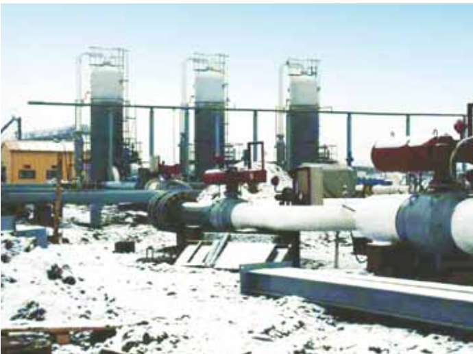
Mogilno underground natural gas storage and above ground gas compressor and treating station, Poland for Polish Oil Gas Co.
