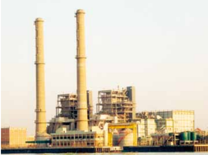
Integrated Power Plant – 320 MW, Congo for ENI Congo S.A.
