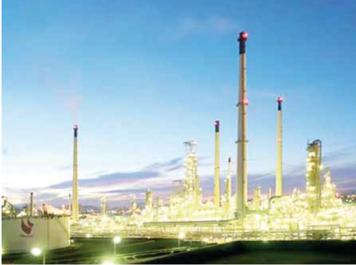
CDU 3 Refinery Revamping Thailand for Thai Oil Ltd
