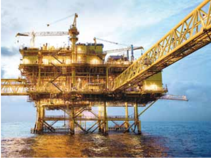
PB-KU-H Production Platform, Mexico for Pemex
