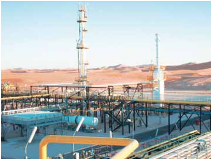
Bir Berkine/Bir Berkine Nord Oil Treatment Plant, Algeria for Sonatrach
