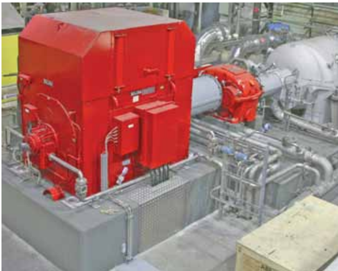
Blast furnace blower motor (8.4 MW) which is controlled by an ACS 5000
