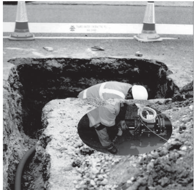
Underground Installation of AquaMaster
