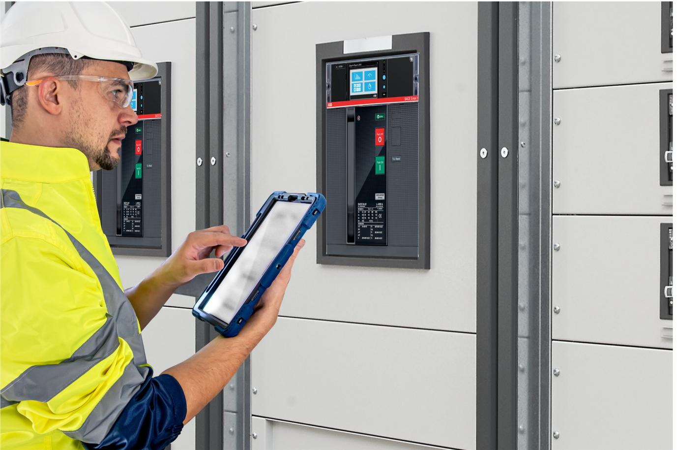
First, it is necessary to establish a connection between Ekip Connect 3 Software and the circuit breaker that needs to record.
