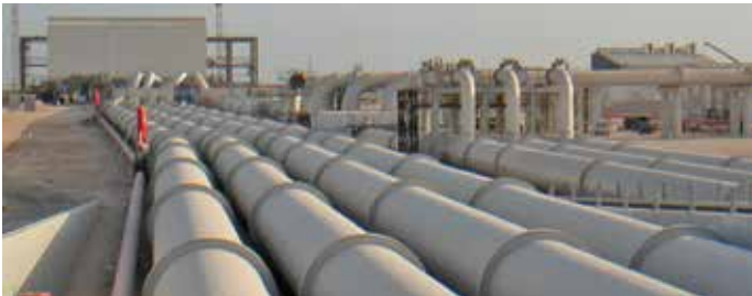
Cooling water supply
