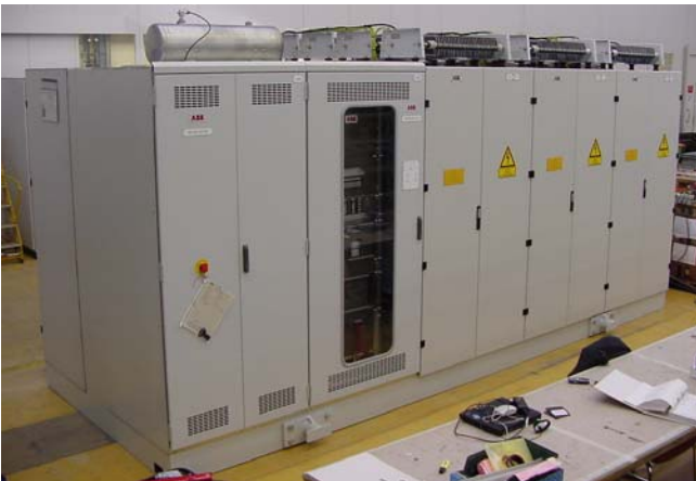
Figure 4: Cycloconverter during testing
