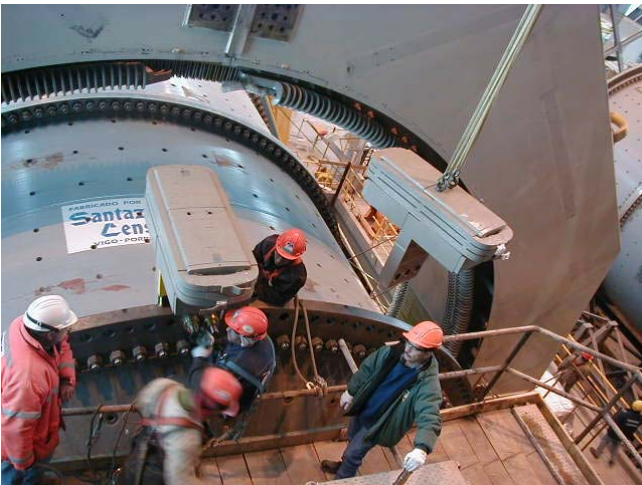
Figure 3. Pole mounting during installation of ringmotor
