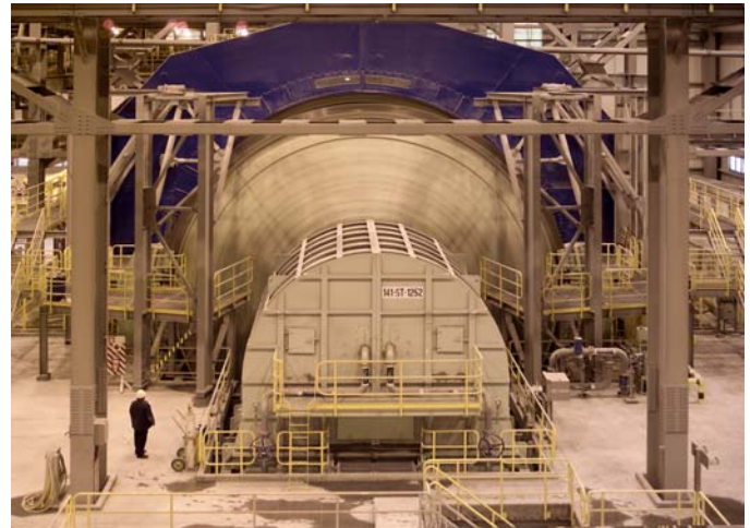
Figure 1. Picture of a typical GMD system for a SAG mill
