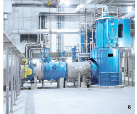
1 Vertical high voltage induction motor rated at 3.5 MW | 2 ACS 1000 variable speed drives rated at 3.5 MW | 3 Variable speed drive supply transformers | 4 Low voltage switchgear | 5 Electromagnetic flowmeter | 6 AMB vertical high voltage induction motor rated at 1.8 MW
