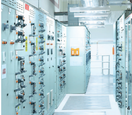
1 Vertical high voltage induction motor rated at 3.5 MW | 2 ACS 1000 variable speed drives rated at 3.5 MW | 3 Variable speed drive supply transformers | 4 Low voltage switchgear | 5 Electromagnetic flowmeter | 6 AMB vertical high voltage induction motor rated at 1.8 MW
