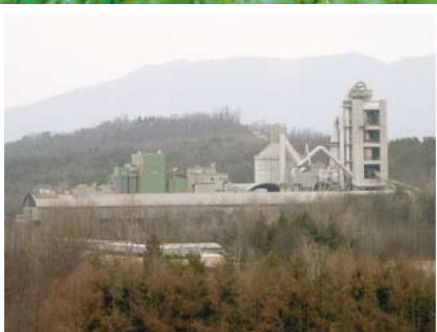
Figure 2. Holcim Ternate plant, Italy, where clinker production was increased by as much as 8% and freetime standard deviation reduced by 25% by the use of the Expert Optimizer.
