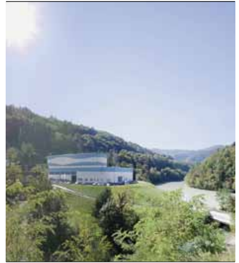
1 The Avče power house located on the Soca river side, looking over the lower reservoir
