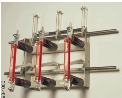
98-1060 Disconnector fitted with earthing knives
