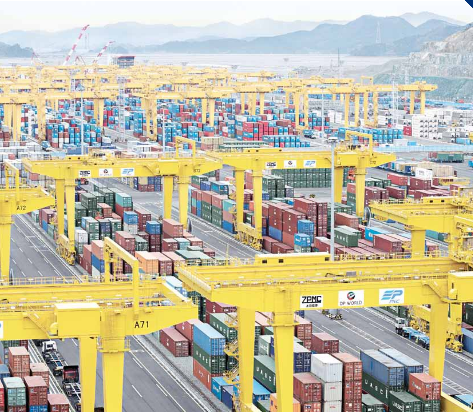
Magnificent view: The impressive fleet of fully automatic stacking cranes at Busan Newport 1-2 Terminal in Korea has been taking care of the yard operations since 2009. The terminal's latest extension opened for operation in 2012.
