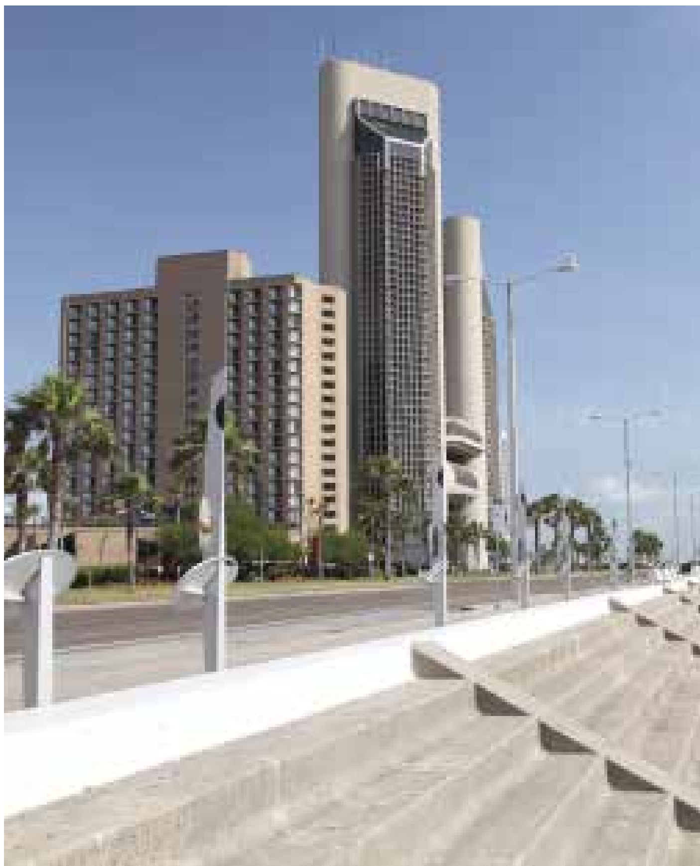
Corpus Christi, Texas, which deployed an automated meter reading (AMR) system for its municipal water and gas utility.
