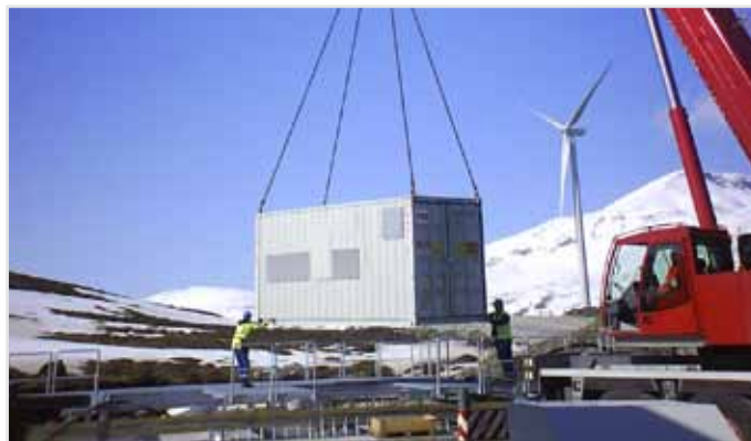
A crane positioning one of the PCS100 STATCOM containers into place
