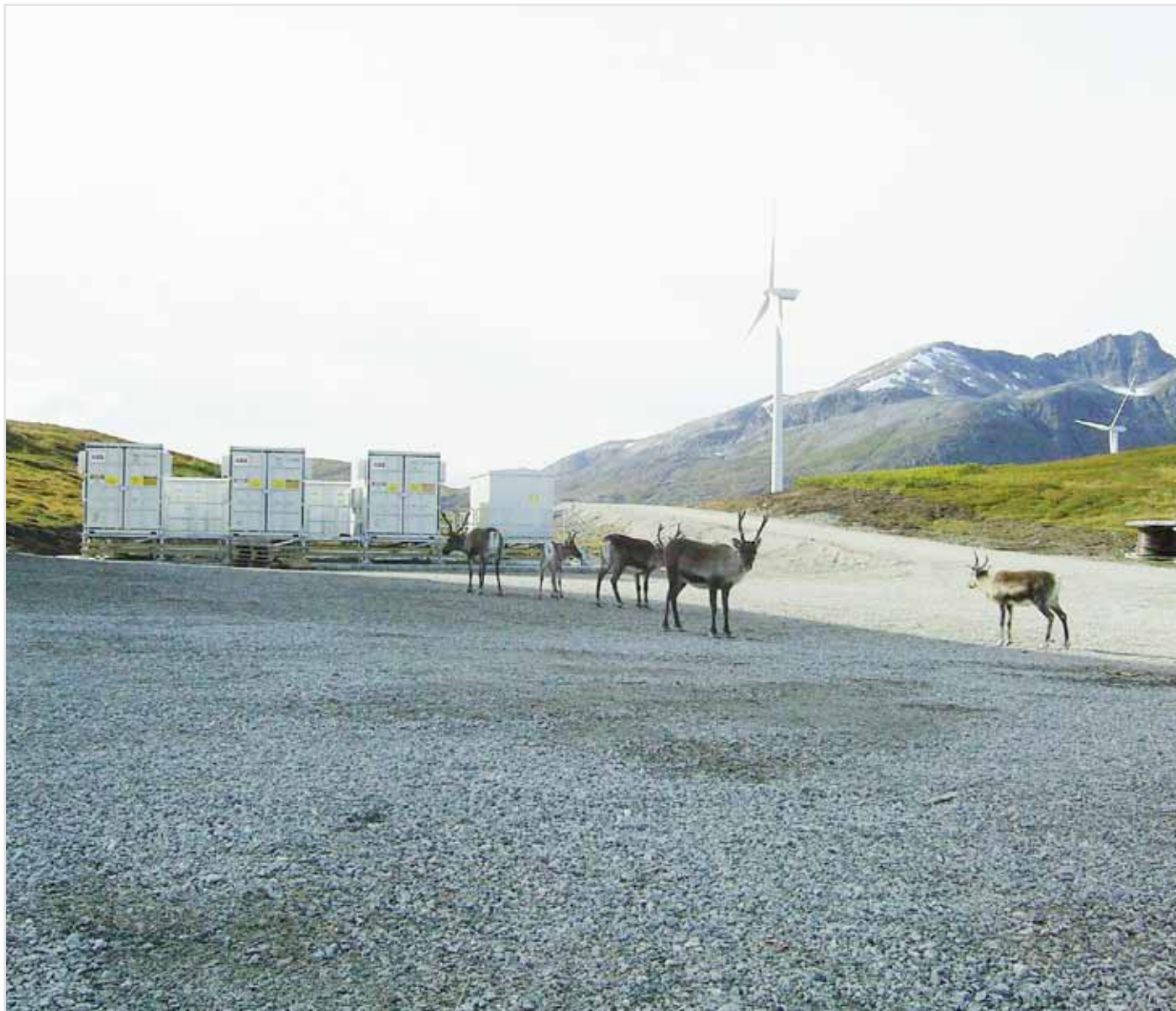
Three 2 MVar PCS100 STATCOM containers for a 54-megawatt onshore wind farm located in Fakken, in the far north of Norway
