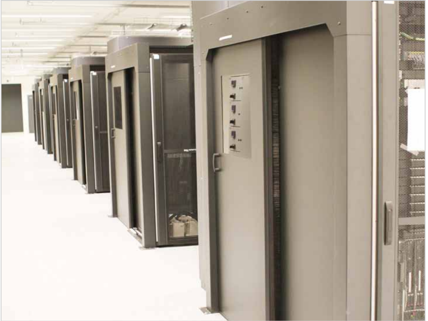
ABB's business partner in Denmark, has delivered a new server room to DONG Energy
