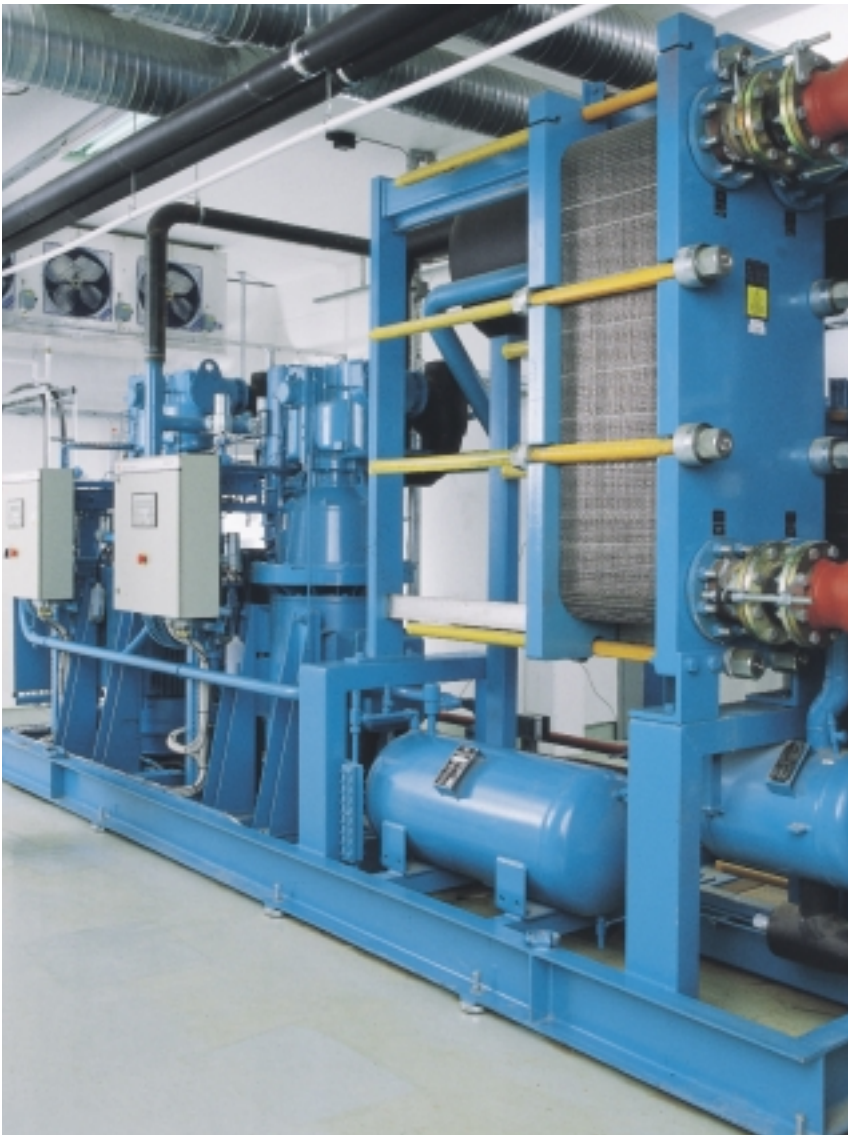
Liquid chiller in a Swedish district cooling system. The unit includes a type FV 26 STAL Rotatune for precise adaptation of capacity to the system load. 9
