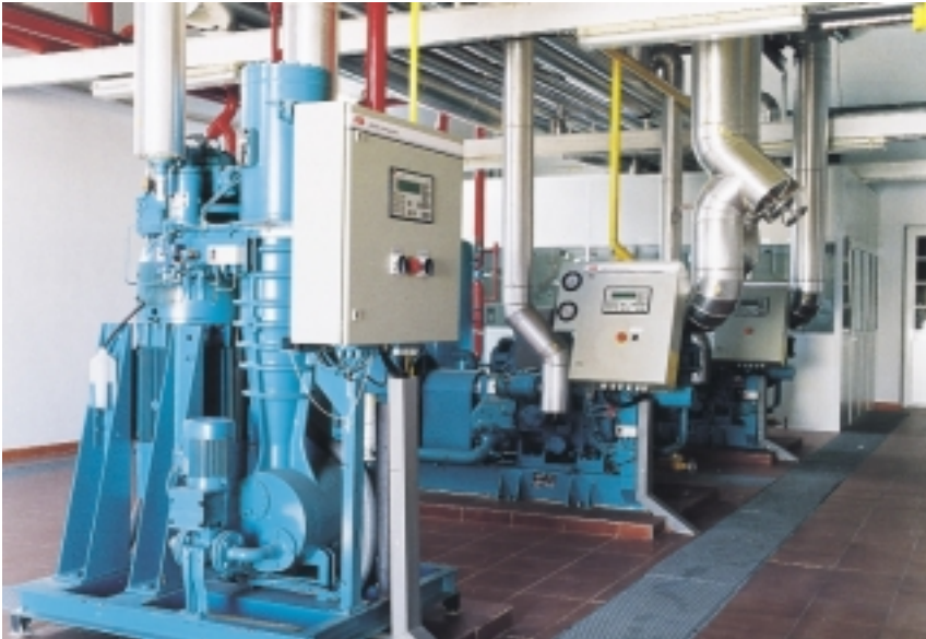
A screw compressor installation for freezing fruit at a Spanish food producer. Capacity control of the plant is provided by a type FV 19 STAL Rotatune unit with economizer.
