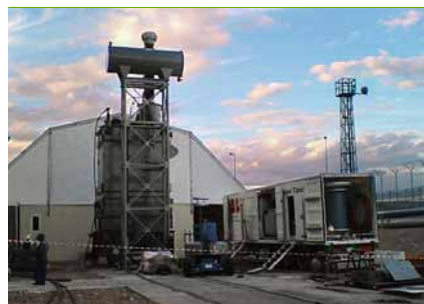
1b A typical set-up for transformer testing at a nuclear power plant
