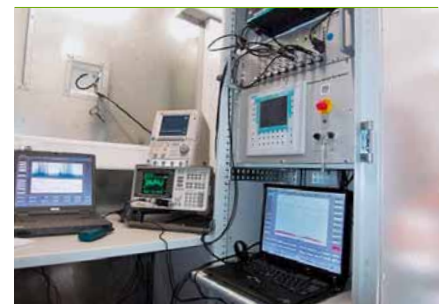
1c Mobile High-Voltage Test System control room
