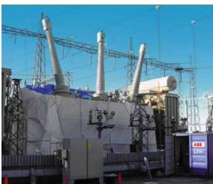
5 On-site drying of a 750MVA/500 kV core type autotransformer with LFH heating combined with hot oil spray
