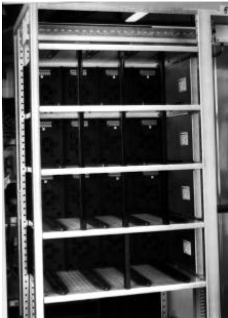
Withdrawable module compartments size 8E/4 and 8E/2
