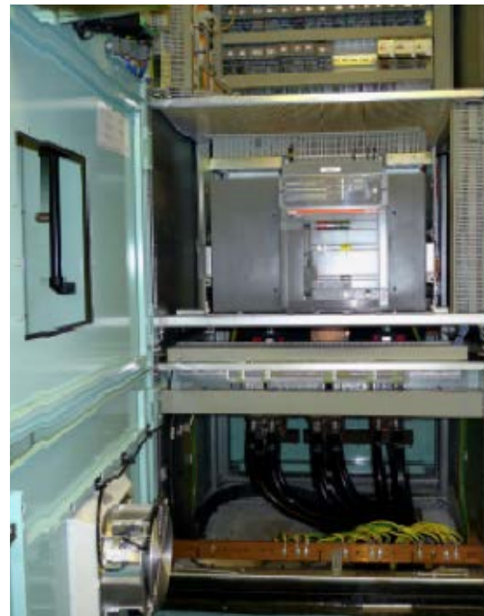
Figure 4: Example of a low voltage shore connection feeder
