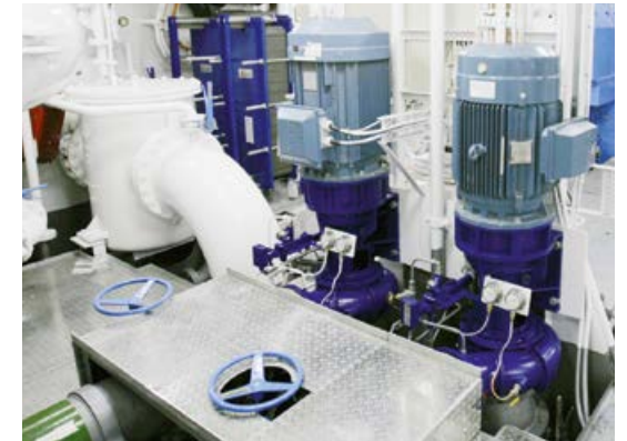
Figure 2: Sea water cooling pumps with ABB high efficiency low voltage motors.
