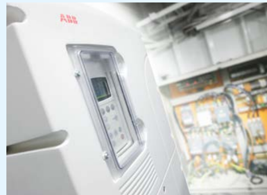
Figure 4: The wall mounted ACS800 industrial drive with built-in winch control program replaced contactors for smooth, trouble free starting.
