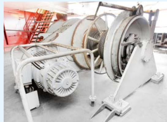
Figure 1: The existing winch motor, motor cable, mechanical disc brake and operator control stand were reused.
