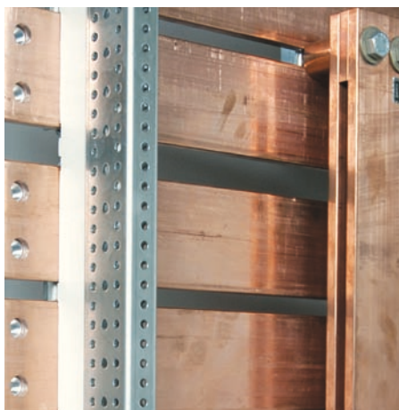
The position of the main busbars increases personal safety and ensures low internal temperatures
