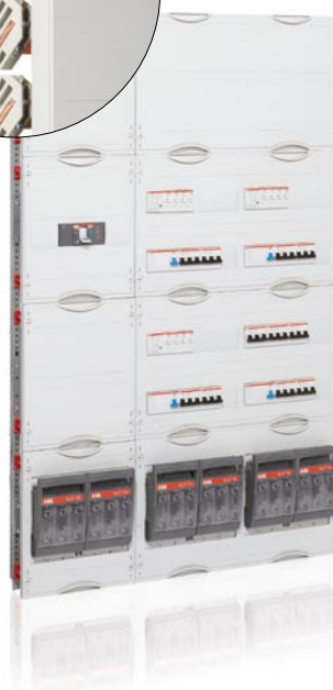
WR mounting frame up to 850 A
