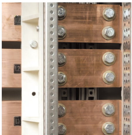
Maintenance-free busbar connections guarantee optimum contacting and thus a high level of safety, availability and economy
