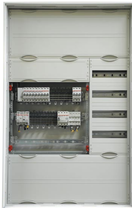
Wall-mounting cabinet fitted with modules on an EDF mounting frame including a module for SMISLINE TP devices with mounting adapter and pro M DIN rail mounting devices.
