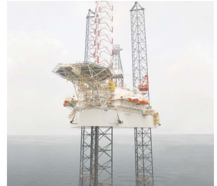
The COSLCraft jack-up drilling rig was delivered from Keppel FELS in 2007 and utilizes a complete ABB electrical solution.
