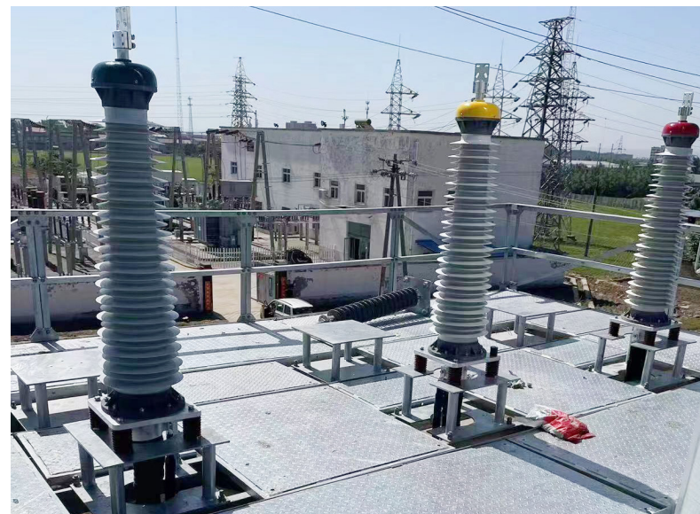
The mounting bracket is of flat structure (Hole spacing 318mm*318mm)
