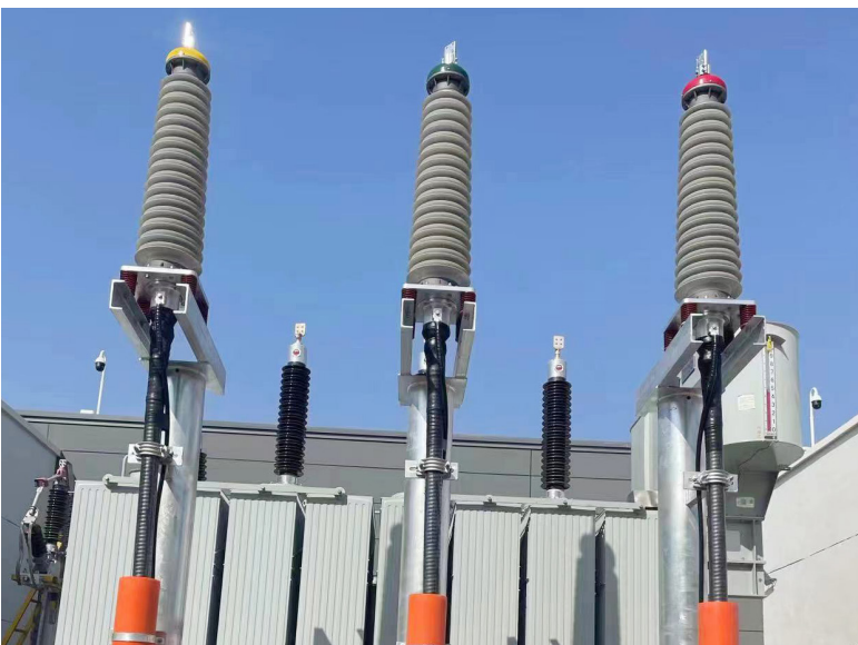
Oil-immersed termination with composite insulator
