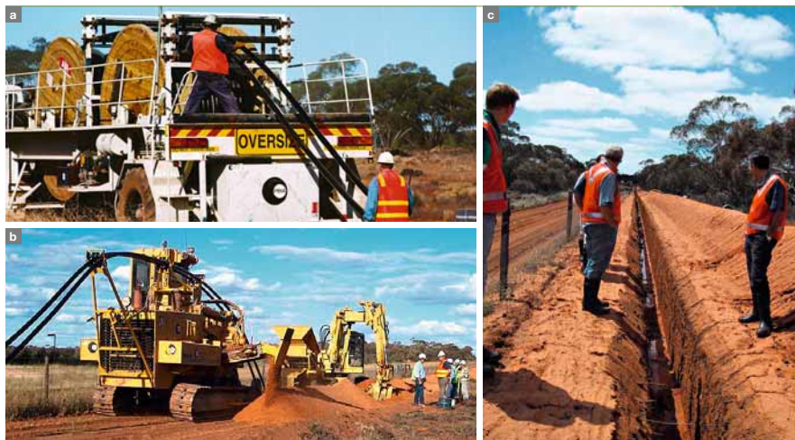
3 Laying HVDC Light® cable in Australia: Transporting the large cable drums a. Preparing to lay the cable using a chain excavator (left) and refilling machine (right) b. A typical narrow cable trench with minimum environmental intrusion c.
