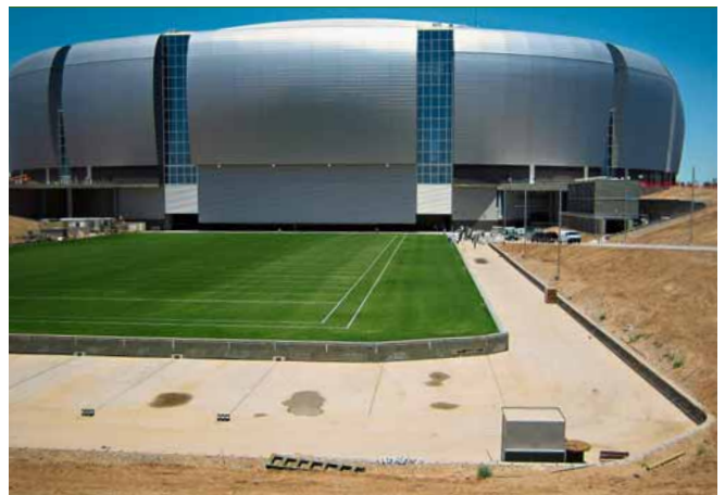
2 The entire playing surface can be rolled out of the stadium.
