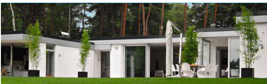
3 Modernized bungalow in Ratingen, Germany
