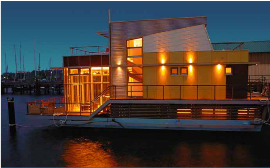
6 The "floating house" pilot project
