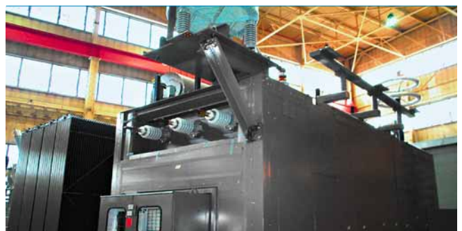
9 Ultra-low noise ConEd transformer with Sound Enclosure
