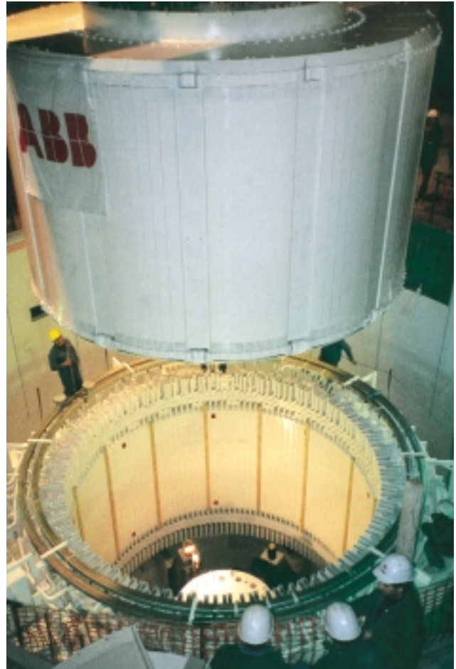
1 Assembling a 465-MVA generator in the cavern of Bieudron hydropower plant. The 454-t heavy rotor has to be lowered into the stator with high precision.
