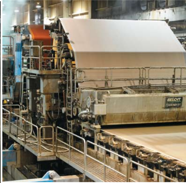
The single 185"-trim fourdrinier board machine with top former—one of the last built by Beloit.
