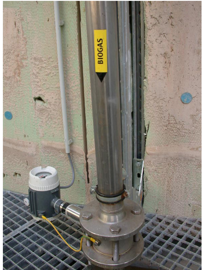
Metering wet gas directly at the secondary fermenter.
