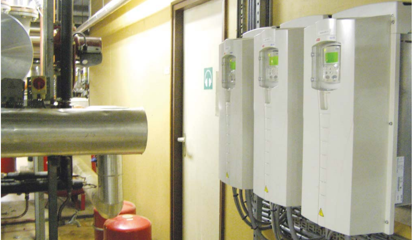
ABB standard drives for HVAC helped to reduce energy consumption by 10%.
