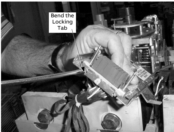
Figure 20. Bending the locking tabs to secure the trip unit plug to the mounting plate.
