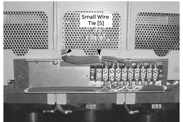
Figure 18. Completed terminal board installation (shown with breaker cover in place).
