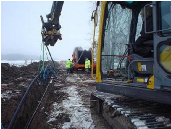
Fig. 6 Land cable laying from a cable wagon.
