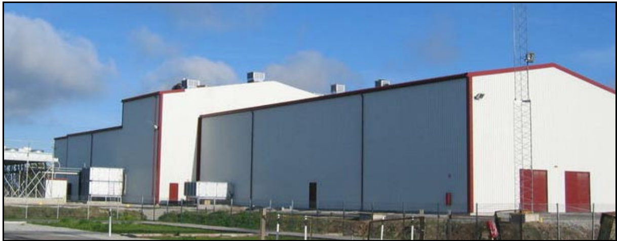
Fig.3 Harku HVDC Light ® converter building
