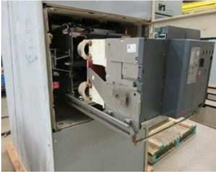
Figure 19. Breaker Positioned on Rails
