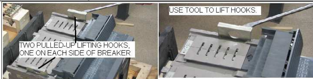
Figure 7. AKD-5—Breaker Lifting Holes
