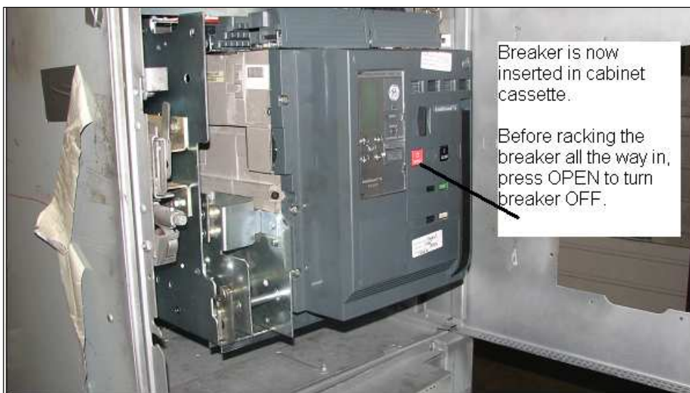
Figure 20. Breaker Ready for Complete Installation
