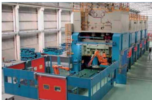
2 An ABB robotic destacker cell in PSA's Poissy factory feeding sheet metal blanks into a press line
